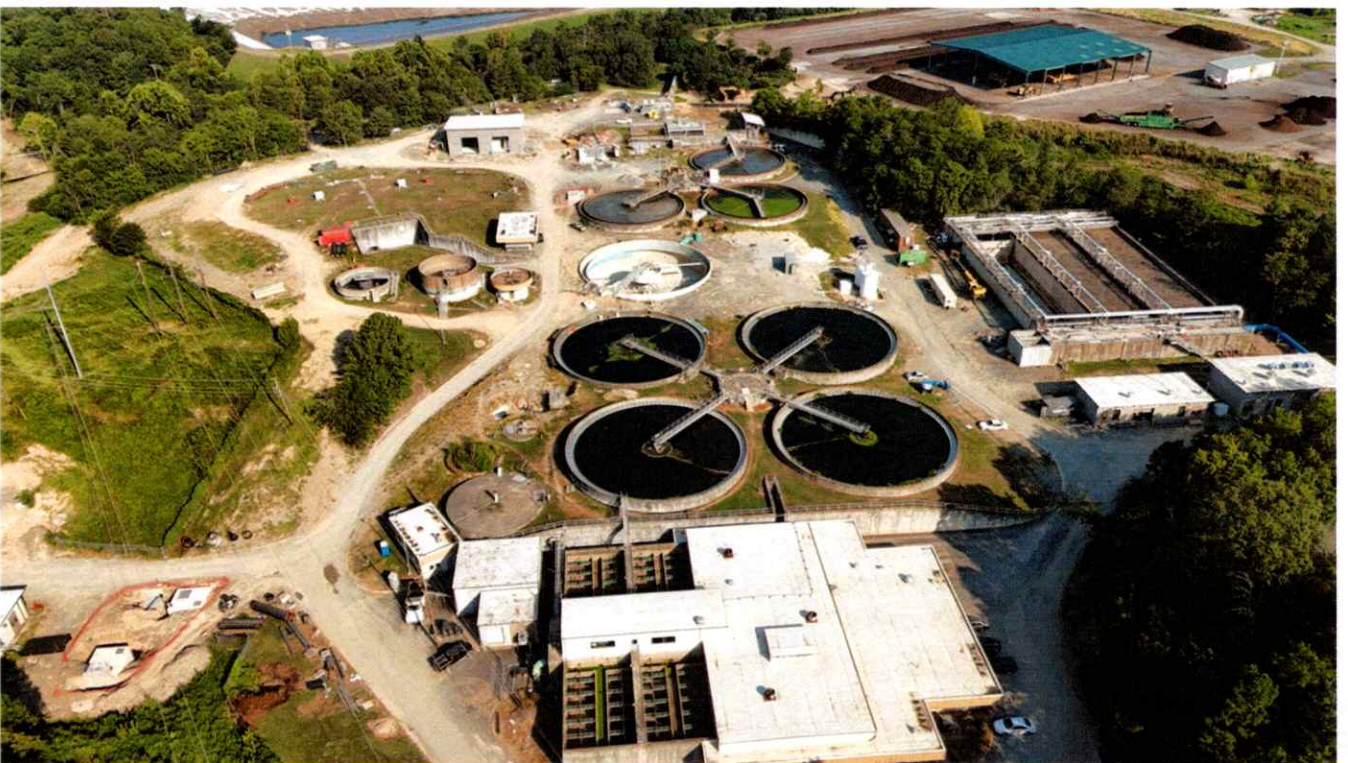
Davidson Drive WWTP Improvements
