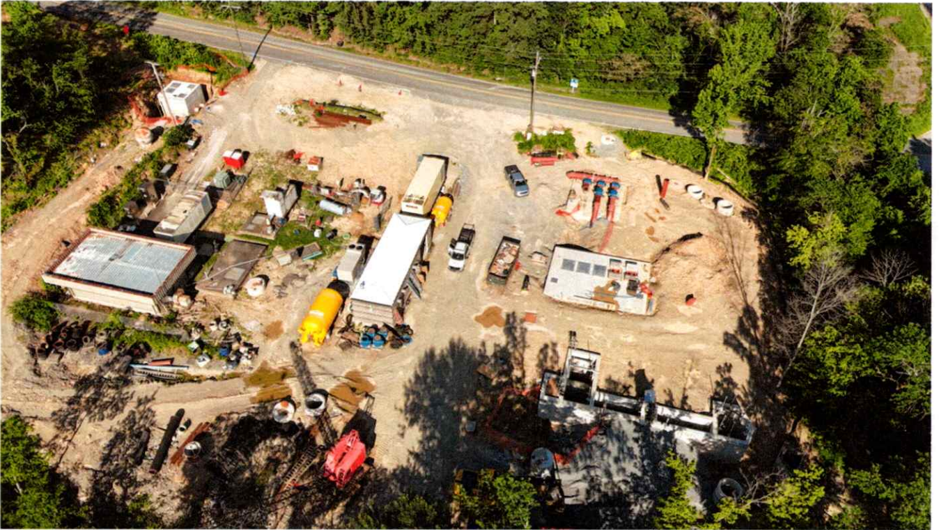
Gulpha Pump Station Improvements
